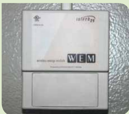
A recently installed wireless energy module, which automatically monitors the heat in apartments and provides residents with consistent, comfortable temperatures.
